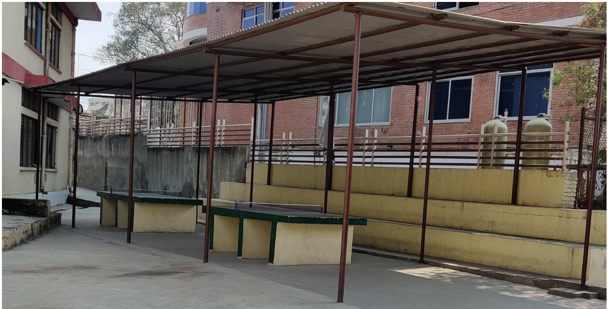
Figure 49: Renovated table tennis court and parapet.
