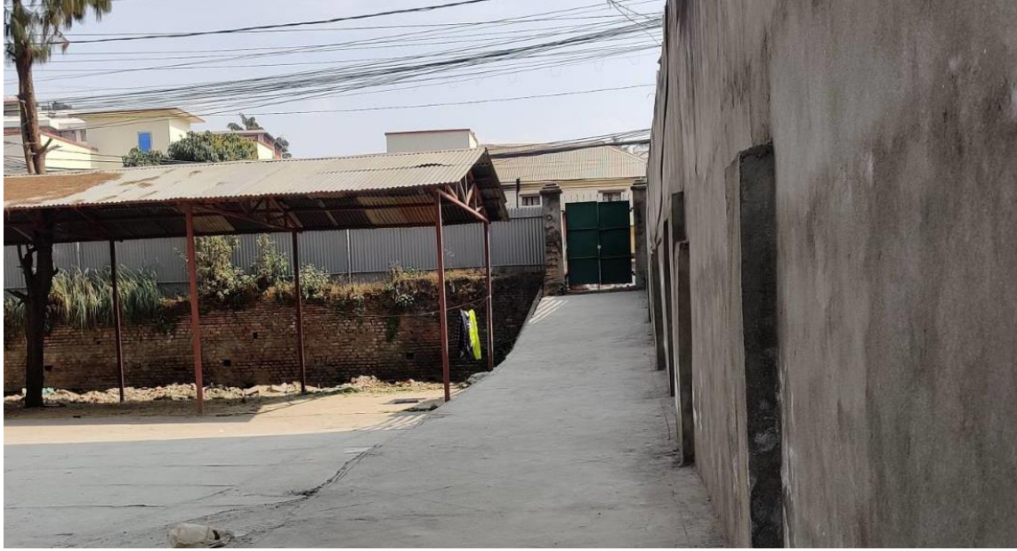
Figure 42: Newly constructed emergency exit
