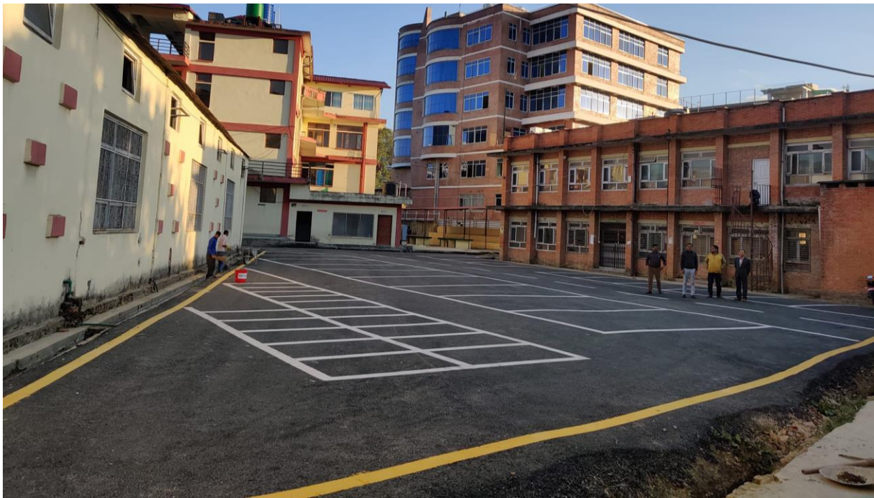
Figure 39: Newly constructed parking space
