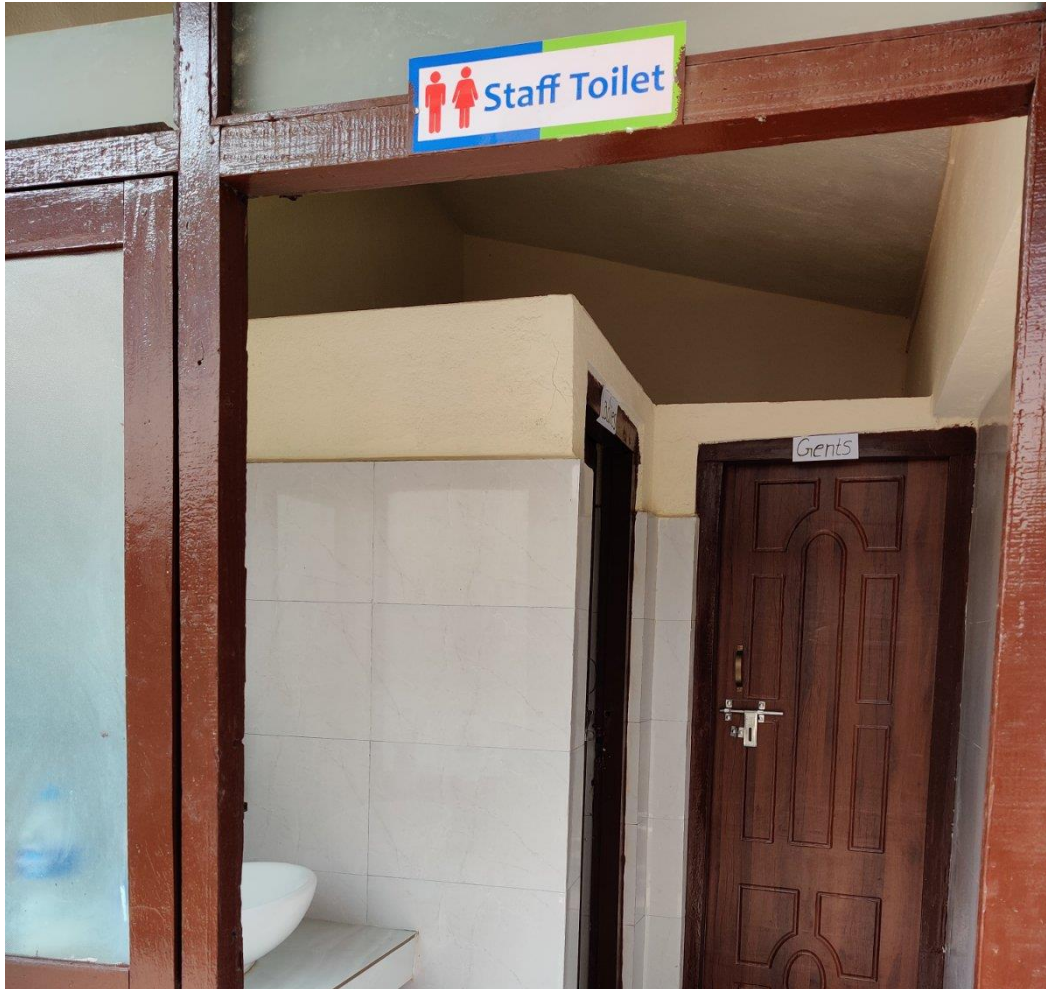
Figure 50: Newly renovated staff toilet.
