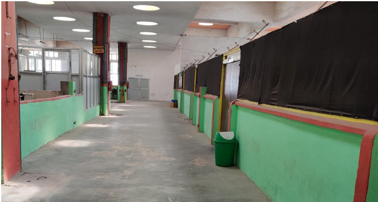
Figure 45: Refurbished Mechanical and Automobile Workshop
